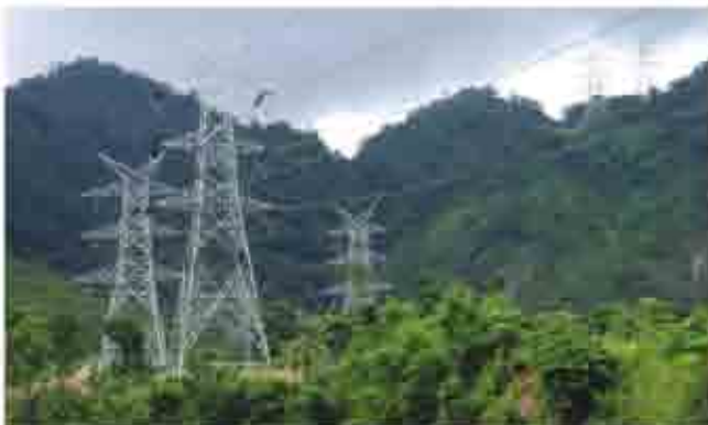
220 KV Transmission line - PGCIL
