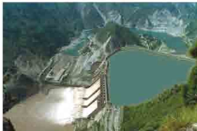
Dam Complex of 690 MW Salal Power Station of NHPC in J&K
